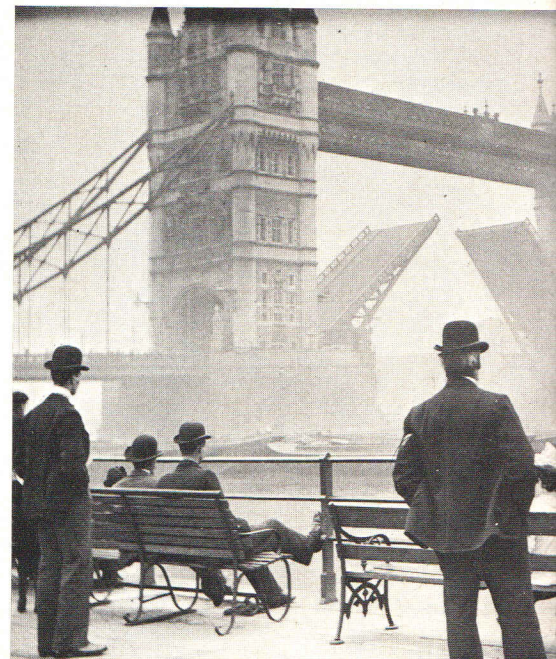
Tower Bridge, a triumph of Victorian engineering, opens its roadway to let a ship pass.
